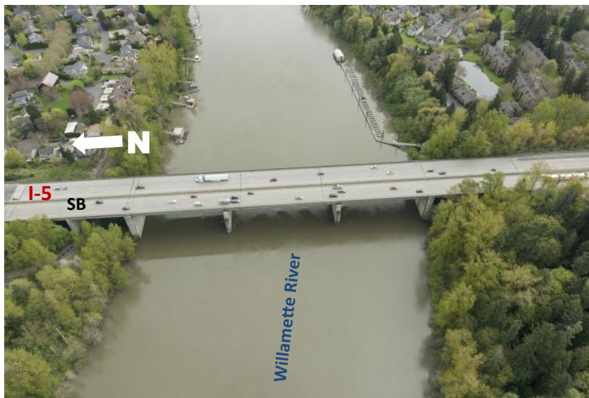
FIGURE 5. I-5 Boone Bridge over the Willamette River.
